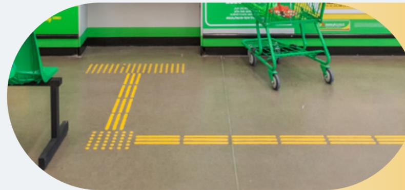
**Podotactile floor:** tactile guides indicating direction and shifts for the visually impaired.
